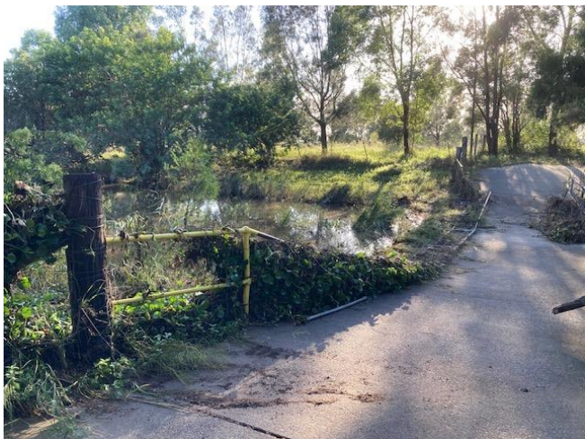
Railings on both sides of the culvert at Snake Gully were flattened.
